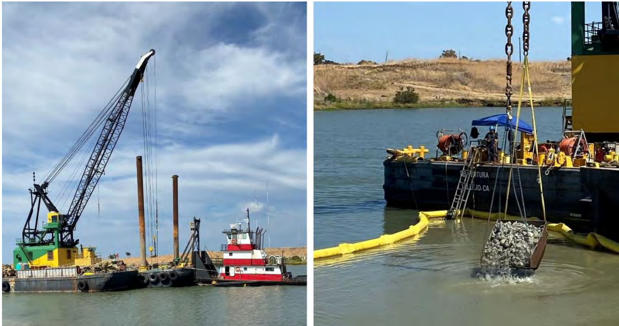
Figure 2-2. Photographs of a Derrick Barge Installing Rock
