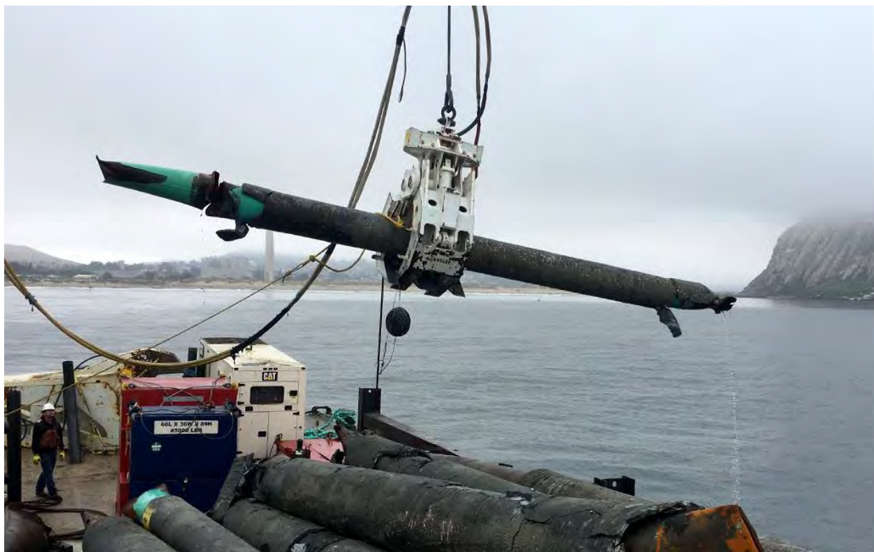
Figure 2-6. Photograph of Pipeline Removal with Crane and Grapple
