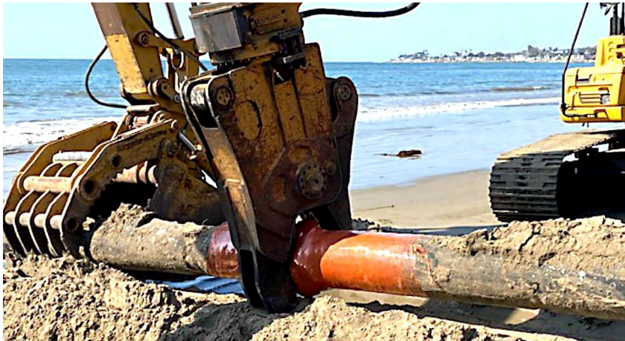
Figure 2-4. Photograph of Pipeline Cutting with Excavator-Mounted Shear
