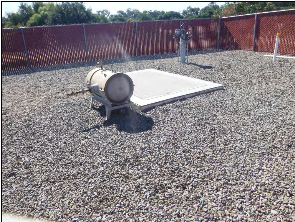
Figure 5-4. Overview of valve vault, facing west
