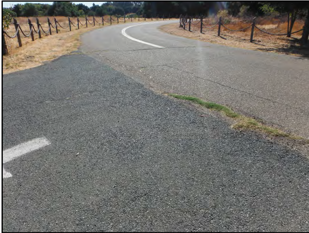
Figure 5-7. Overview of access road, facing west
