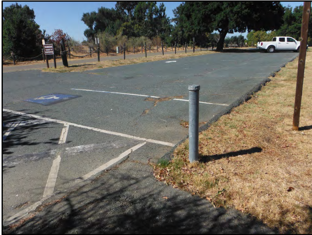
Figure 5-1. Overview of parking lot, facing northeast
