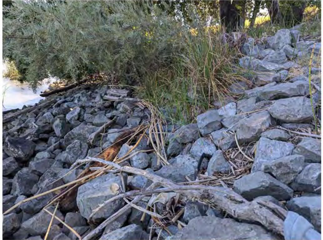
Photograph E. View of the south bank of Threemile Slough along the waterside slope of the Sherman Island levee showing drift deposit where the high tide line was mapped. View northeast (photograph taken 8/15/24).
