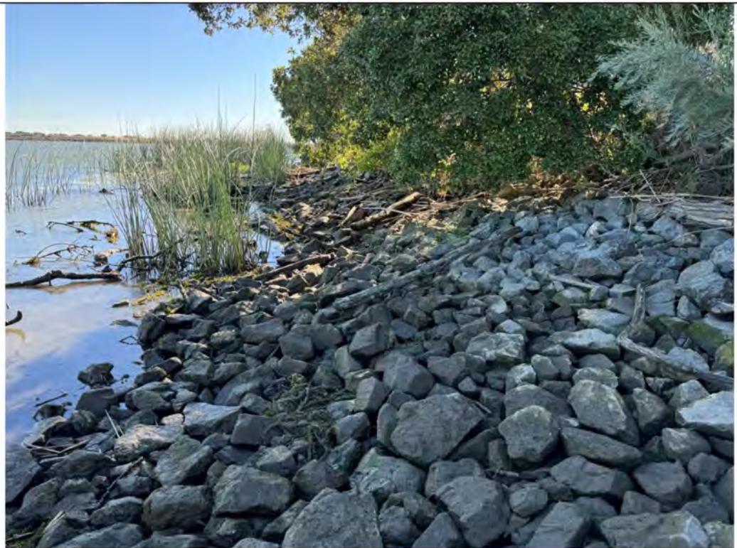
Photograph B. View of the south bank of Threemile Slough. Photo shows rip rap along the waterside slope of the Sherman Island levee. View northeast (photograph taken 8/15/24).
