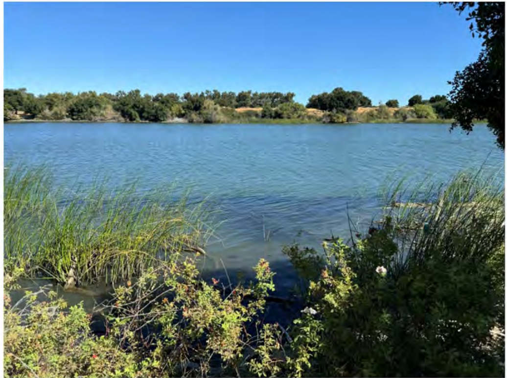
Photograph A. View across Threemile Slough where the pipelines will be decommissioned, taken from the southern bank on Sherman Island. View northwest (photograph taken 8/15/24).
