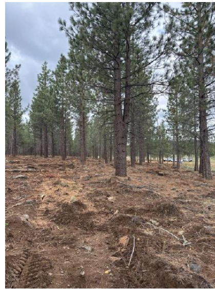
Prosser Dam Project (Zone 3) After Treatment, May 2026
