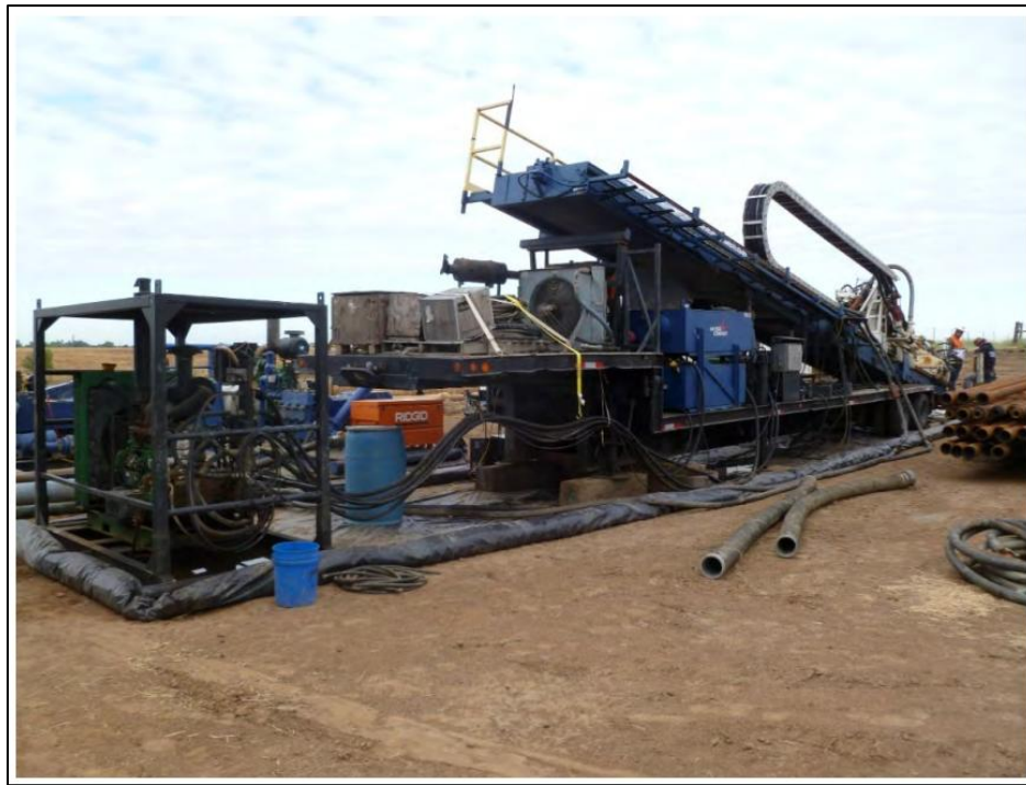
Figure 2-7. HDD Drill Rig
