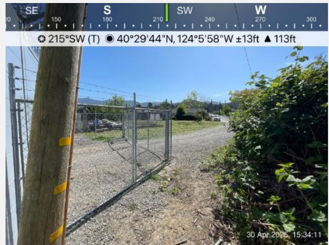
Photo 34. Entrance to substation at southern end of BSA, facing southwest.
