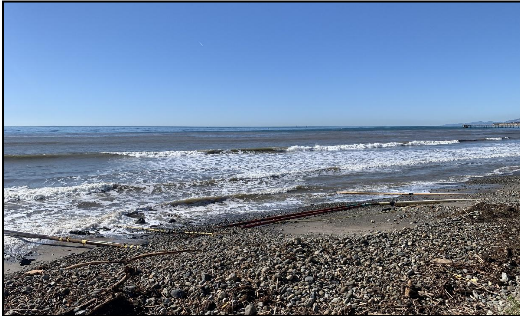
Figure 7. Platform Holly Pipelines Exposed at Haskell's Beach (Winter Conditions – January 2023)
