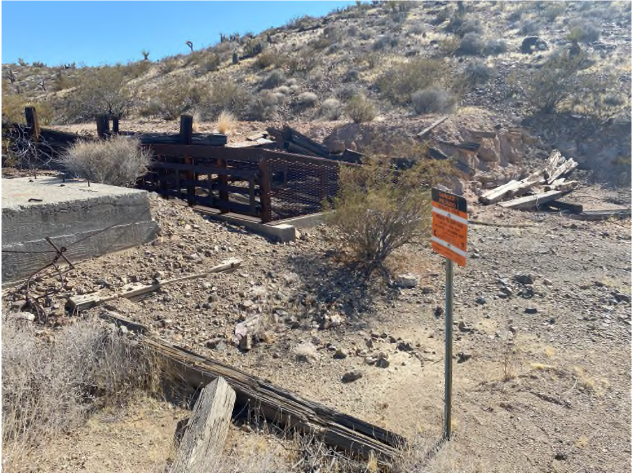
Figure 9: Cupola installed on an abandoned mine shaft.
