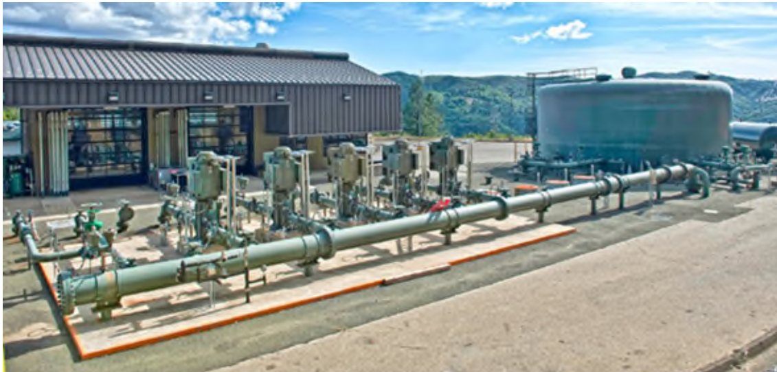
Figure 3: Santa Rosa Geysers Recharge Project, one of two large-scale recycled water injection projects at The Geysers, delivers and distributes approximately 11 million gallons of recycled water daily. Photo by John Grice courtesy of the © 2025 Calpine Corporation. All Rights Reserved.
