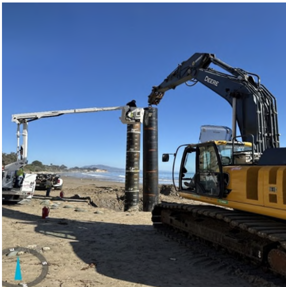
Well A 24-inch casing Installation.
