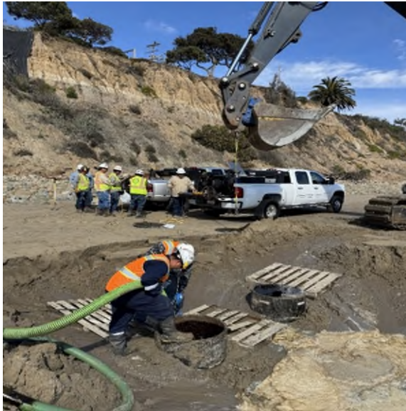
Well A suction operation in progress before installation of well cap.
