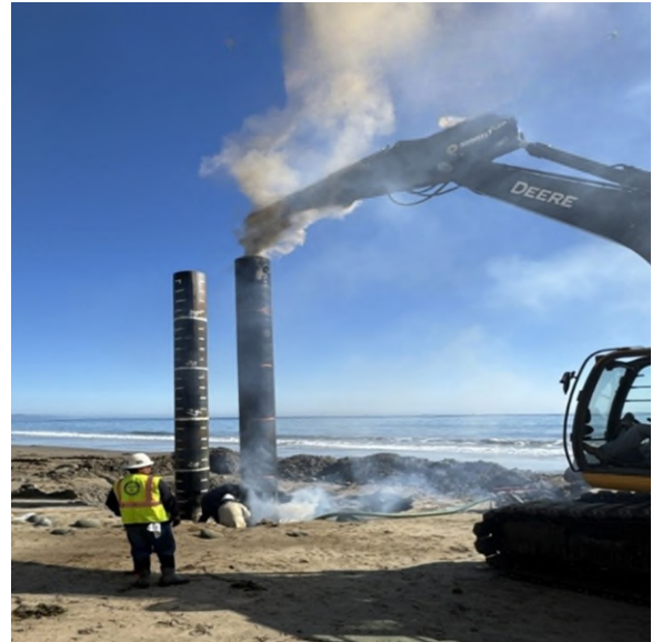
Cutting off excess casing on both Wells A and B.
