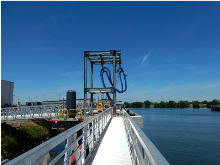
New BWC Stockton Berth 8 Marine Oil Terminal with hose tower for transfer operations
