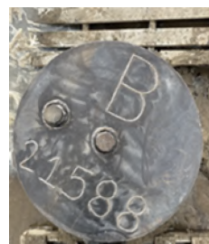
Figure 4. Final welded well abandonment plates with API numbers. Photo credits: 2H Offshore
