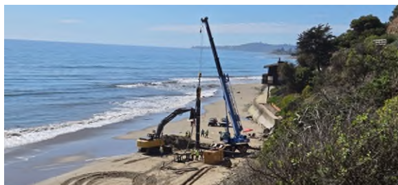
Figure 1. Aerial view of pipe pile installation taken from Lookout Park.
