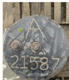
Figure 2. Final welded well abandonment plates with API numbers.
