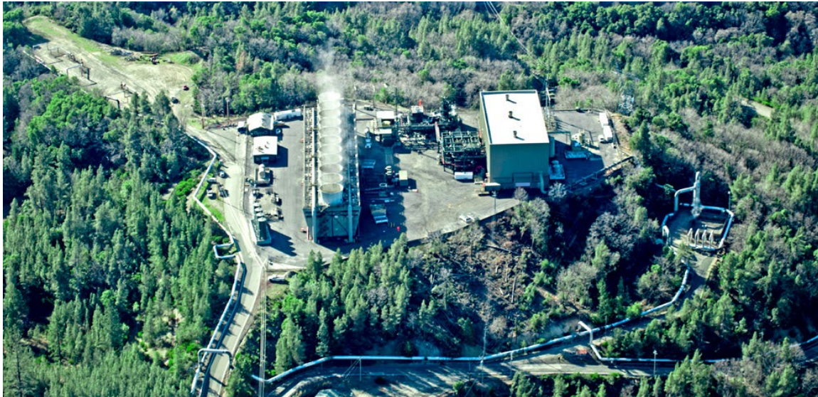
Figure 2: Calpine's Socrates Unit 18 power plant at The Geysers. Photo by John Grice, courtesy of the Calpine Corporation.
