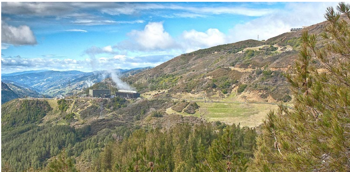
Figure 1: Calpine's Geysers Unit 20 power plant at The Geysers. Photo by John Grice, courtesy of the Calpine Corporation.
