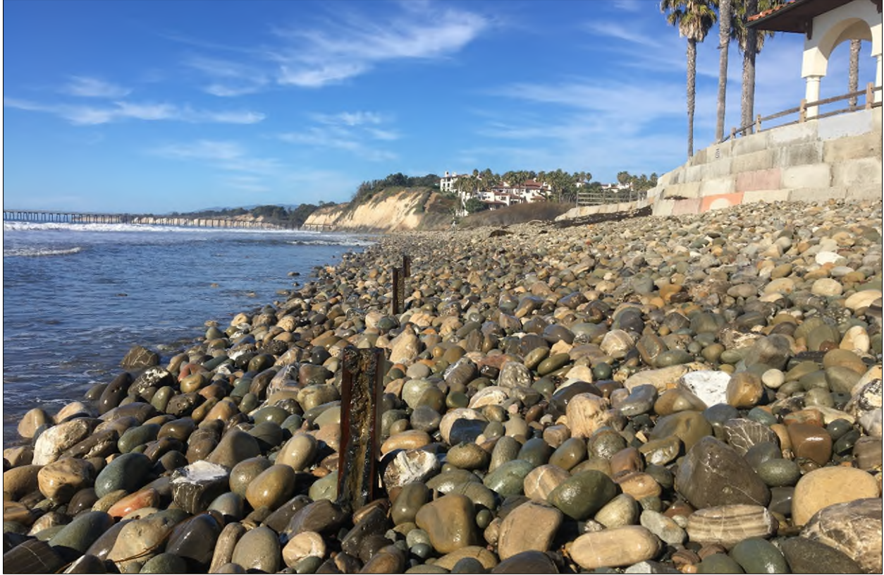
Figure 2. Exposed railroad irons near Goleta Beach (photo by Padre Associates).
