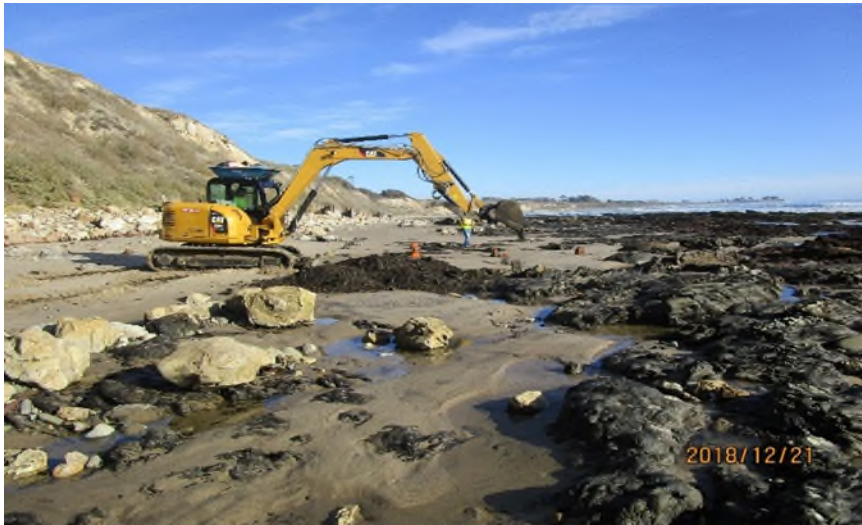
Figure 2. Removal of exposed H-beams from the beach. Photo by Commission staff.
