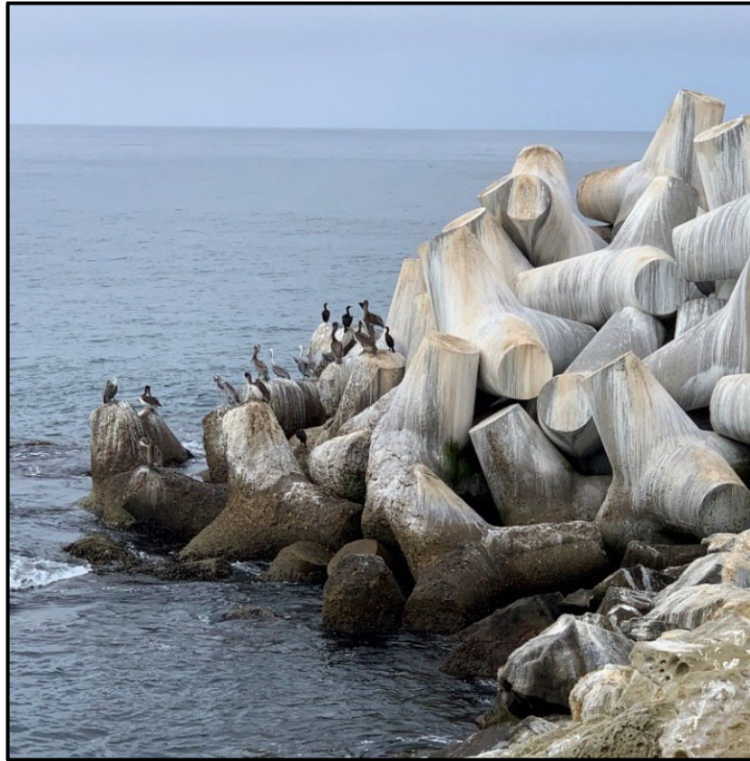
Figure 2-2. Concrete Tetrapods
