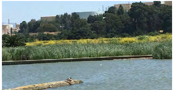
Breakwater Section E - Section not inspected due to shallow water depth
