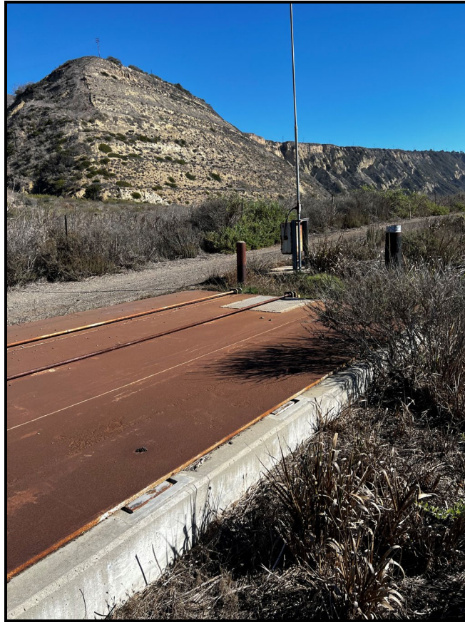
Figure 4.3-6. Onshore Pipeline Connections Vault Box
