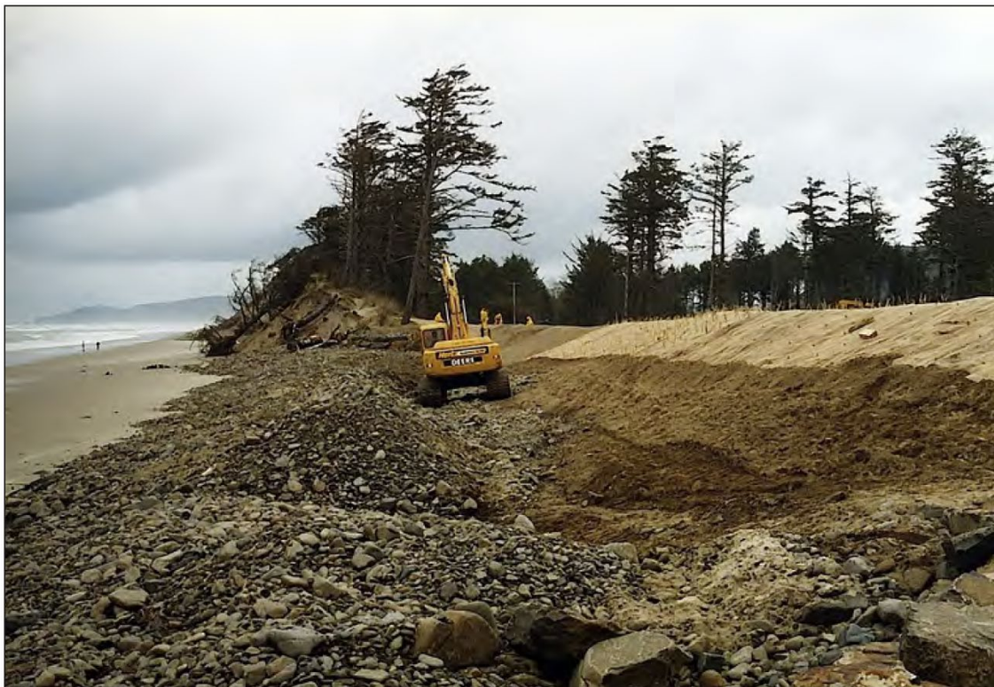
Figure 21. Cape Lookout State Park cobble berm under construction (from Komar and Allan, 2009)
