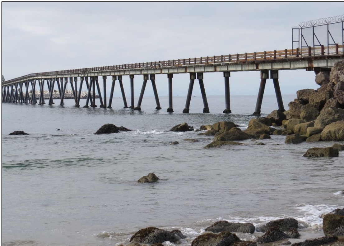
Figure 29. View of the causeway from downcoast showing wide spacing and small diameter of pilings.
