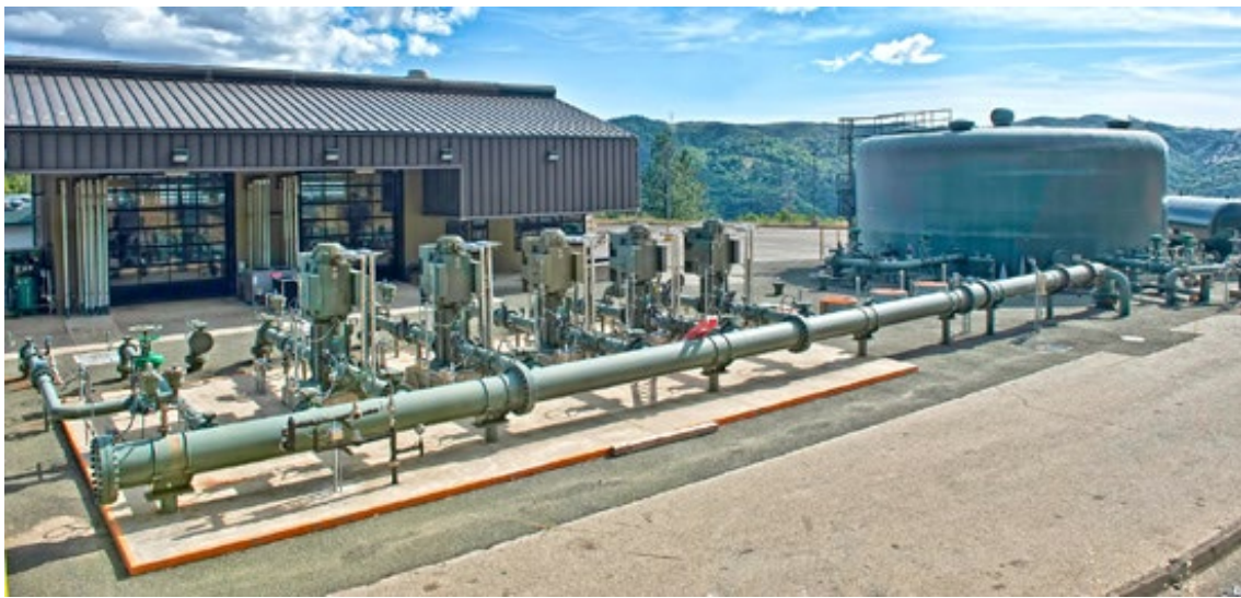
Figure 3: Santa Rosa Geysers Recharge Project, one of two large-scale recycled water injection projects at The Geysers, delivers and distributes approximately 11 million gallons of recycled water daily. Photo by John Grice, courtesy of the Calpine Corporation.
