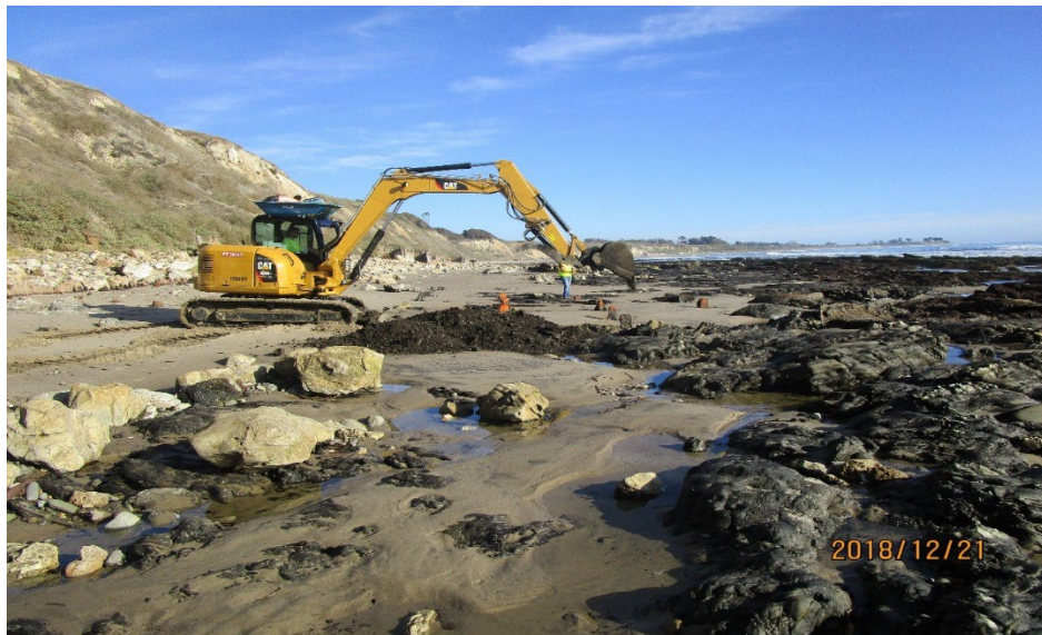
Figure 2. Removal of exposed H-beams from the beach. Photo courtesy of Commission staff.
