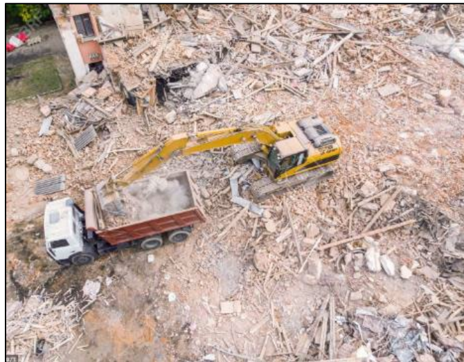
Figure 4.6 | Removal of Rubble Material
