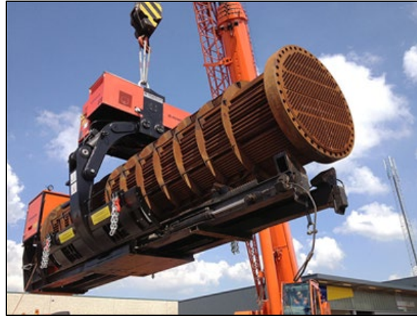
Figure 4.3 | Static Equipment Decommissioning
