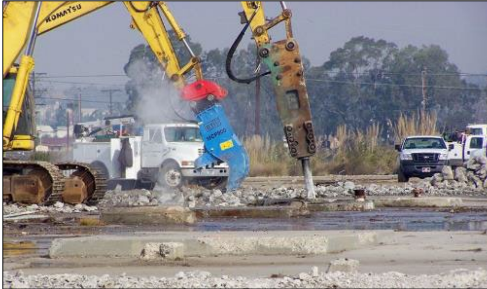
Figure 4.2 | Foundation Demolition
