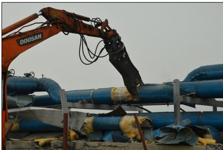
Figure 4.4 | Pipe Sectioning
