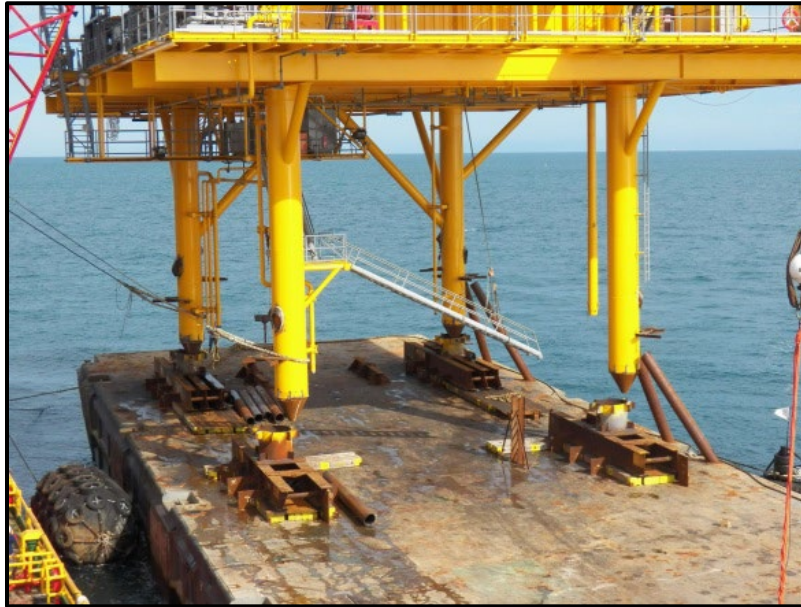
Figure 3.2 | Setting Deck on Cargo Barge
