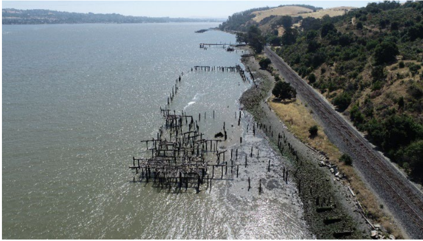
Figure 3. Before photo of Eckley Pier taken July 20, 2023. Photo courtesy of CA State Lands Commission GIS Team
