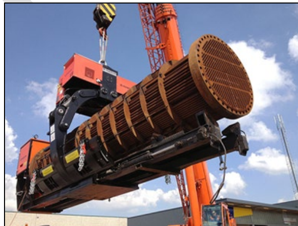
Figure 4.3 | Static Equipment Decommissioning
