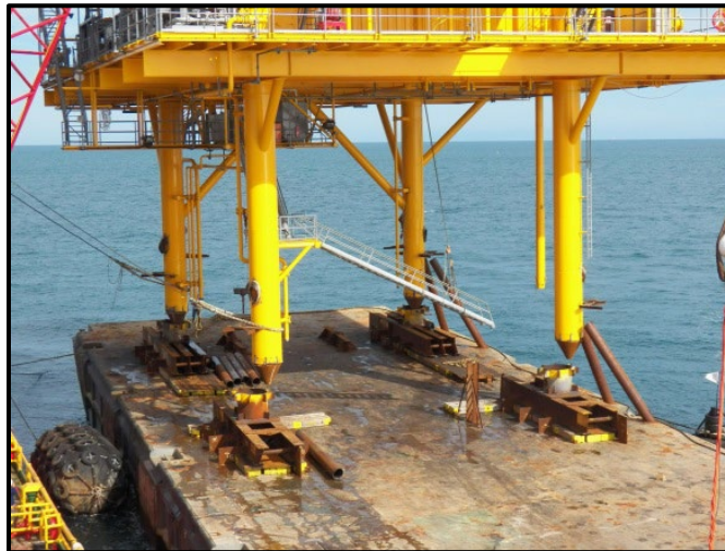
Figure 3.2 | Setting Deck on Cargo Barge
