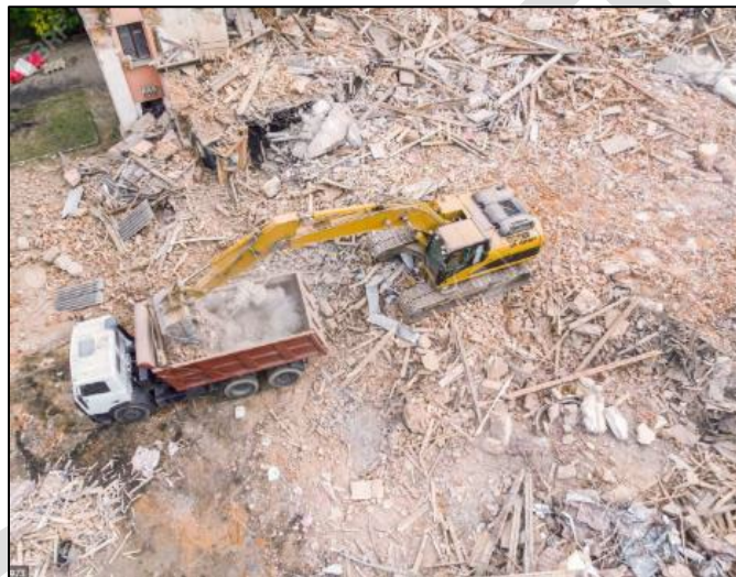
Figure 4.6 | Removal of Rubble Material
