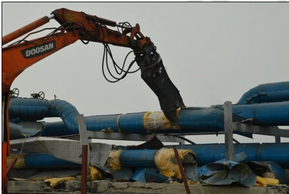
Figure 4.4 | Pipe Sectioning
