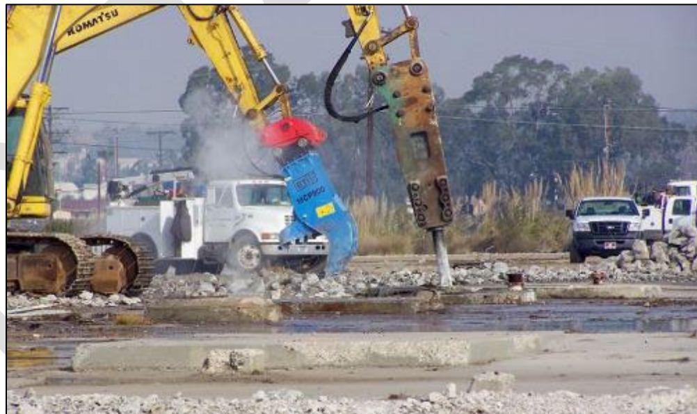
Figure 4.2 | Foundation Demolition
