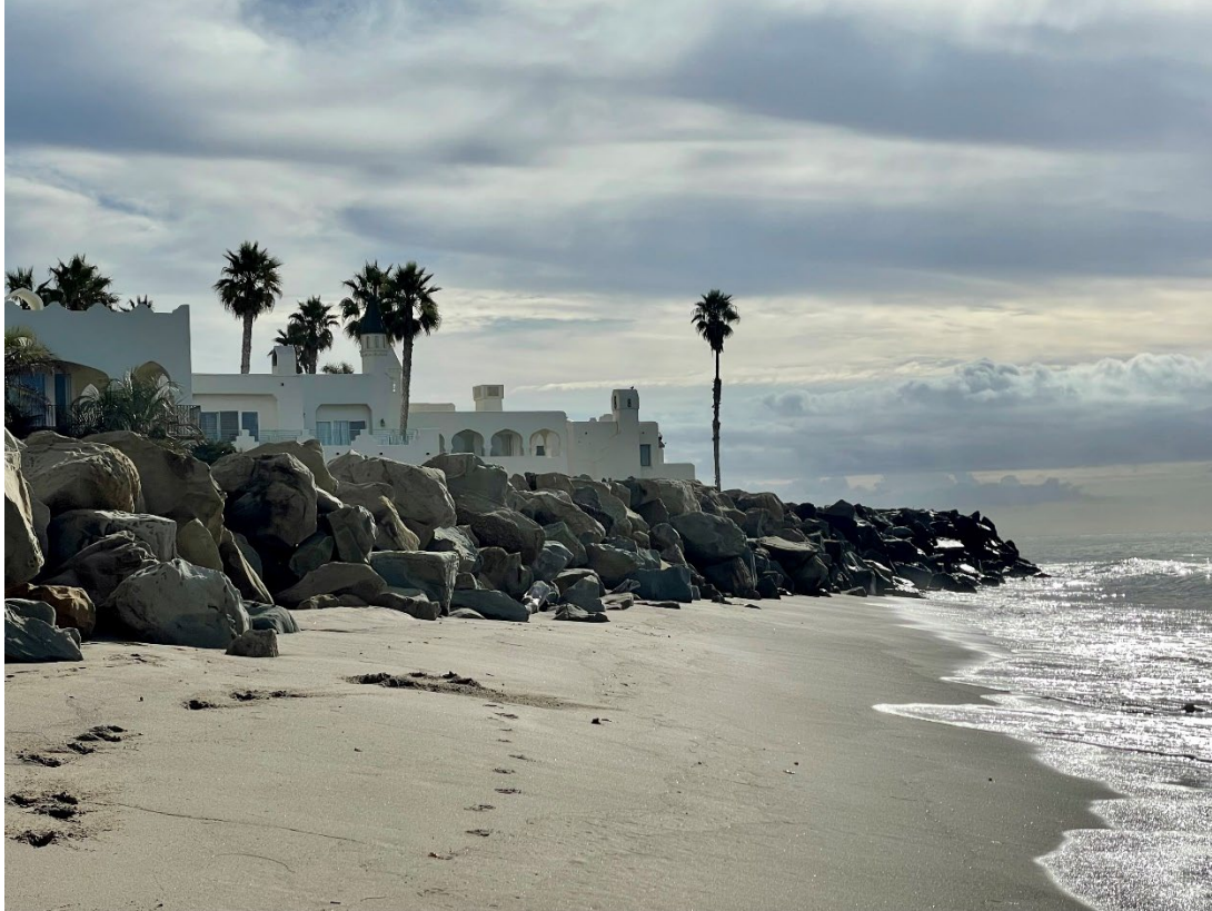
Figure 6: A revetment, used to protect private residential homes in Carpinteria, blocks lateral beach access between Santa Claus Beach and Sandyland Beach. Sandyland Beach cannot be accessed by the public during medium and high tides. Photo: Michael Wells
