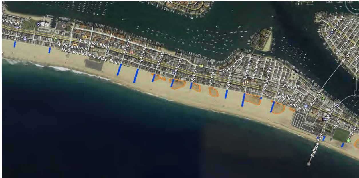
Exhibit 1 , showing in dark blue the locations of 14 walkways that extend through dune and/or beach habitats, between 18 th Street and B Street. Areas of coastal dunes, or potential dunes, are indicated in tan screen. Source: Google Earth Pro.
