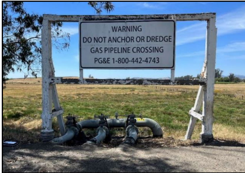
Figure 2-17. Photograph of the Pipe Manifold and Concrete Valve Box on the East Side of Segment 2
