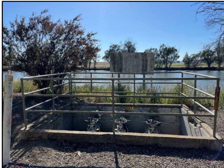
Figure 2-17. Photograph of the Pipe Manifold and Concrete Valve Box on the East Side of Segment 2
