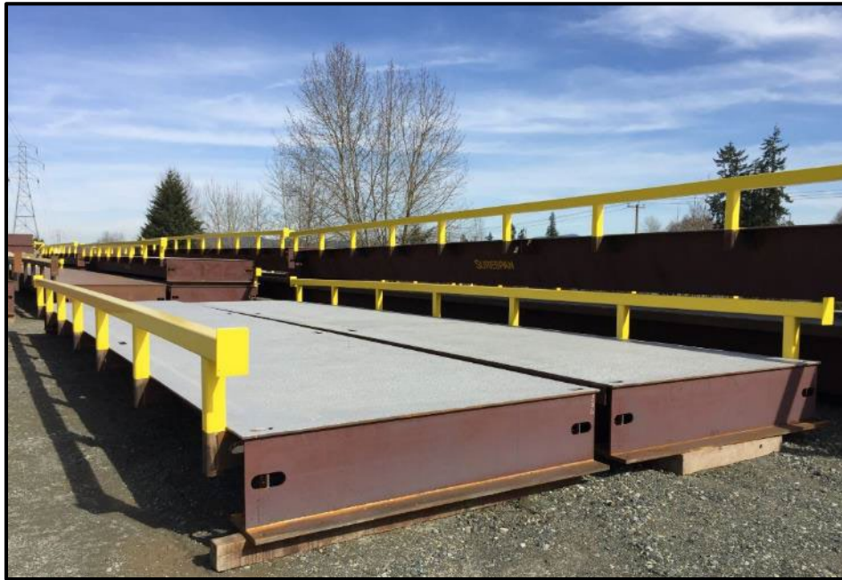
Figure 2-9. Example of a Temporary Bridge
