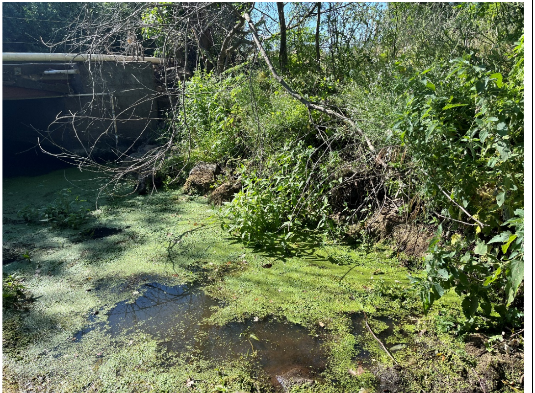
Photograph D. Southeast view of Suscol Creek at the approximate pipeline crossing location. Pipeline will be installed using trenchless installation methods under Suscol Creek. This vegetation community type is defined as an arroyo willow thicket. (photo taken May 24, 2022)
