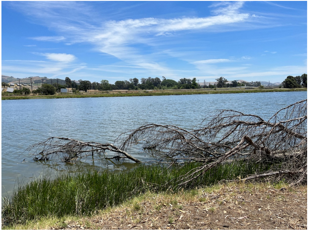
Photograph I. Southeast view of HDD alignment at the river crossing location from the west bank of the Napa River (photo taken May 25, 2022)
