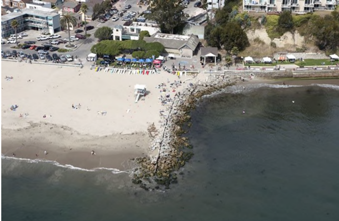
Figure 9: Groin at Capitola Beach. Credit: Copyright (C) 2002-2023, Kenneth & Gabrielle Adelman, California Coastal Records Project, www.Californiacoastline.org
