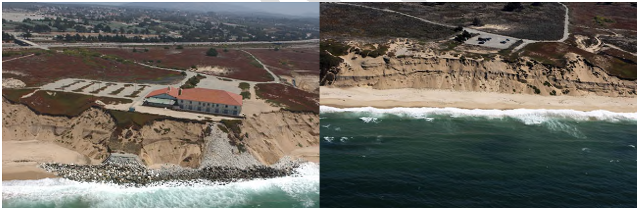
Figure 12: Before (left) and after (right) the removal of Stilwell Hall and a rock revetment at Fort Ord. Credit: Copyright (C) 2002-2023, Kenneth & Gabrielle Adelman, California Coastal Records Project, www.Californiacoastline.org
