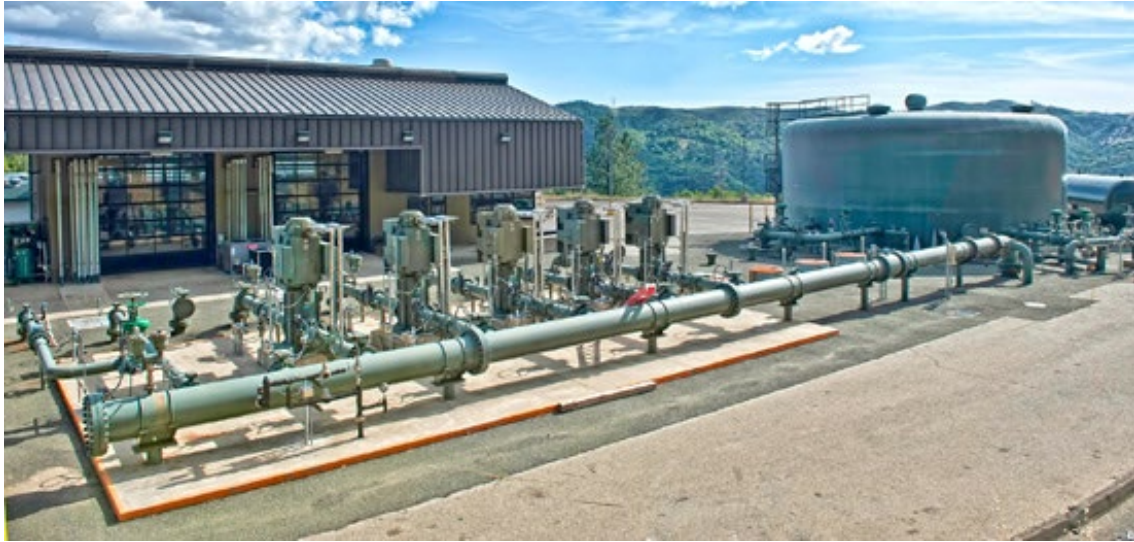
Figure 3: Santa Rosa Geysers Recharge Project, one of two large-scale recycled water injection projects at The Geysers, delivers and distributes approximately 11 million gallons of recycled water daily. Photo by John Grice, courtesy of Calpine.
