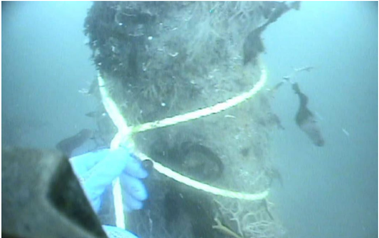
Figure 12. Diver securing travel line along the wells on the Treadwell Pier (photo by Global Diving)
