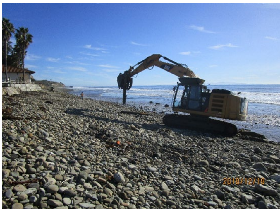
Figure 20. H Beam being extracted near Bacara Resort in 2018 (photo by SLC).
