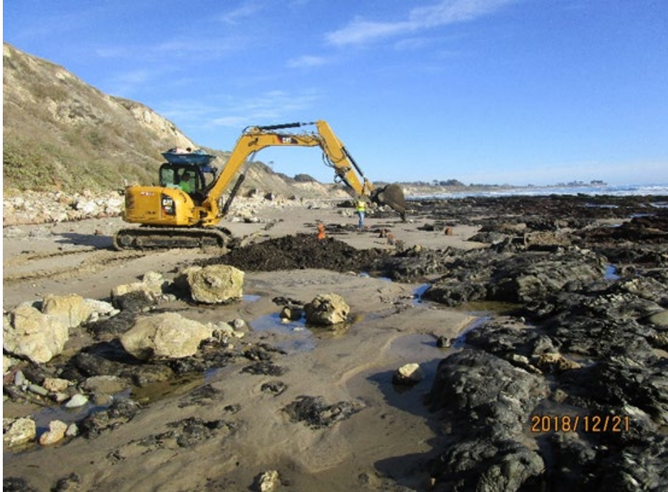
Figure 21. H Beam being extracted near the Bacara Resort in 2018 (photo by State Lands Commission).
