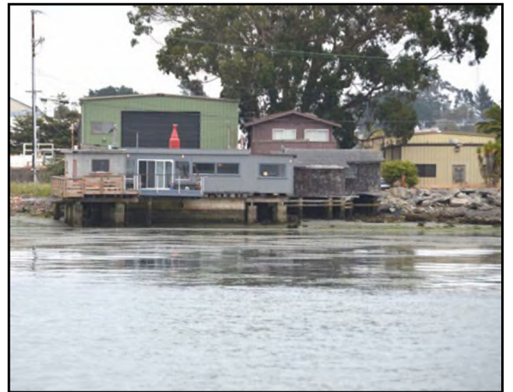
Figure 15 from Humboldt Bay Shoreline Inventory, Mapping and Sea Level Rise Vulnerability Assessment. Building on Eureka Bay. Photo: A. Laird.
