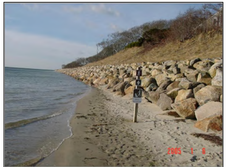
Loss of beach access due to revetments
