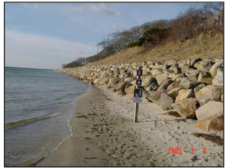
Figure 3 Loss of beach access due to revetments
