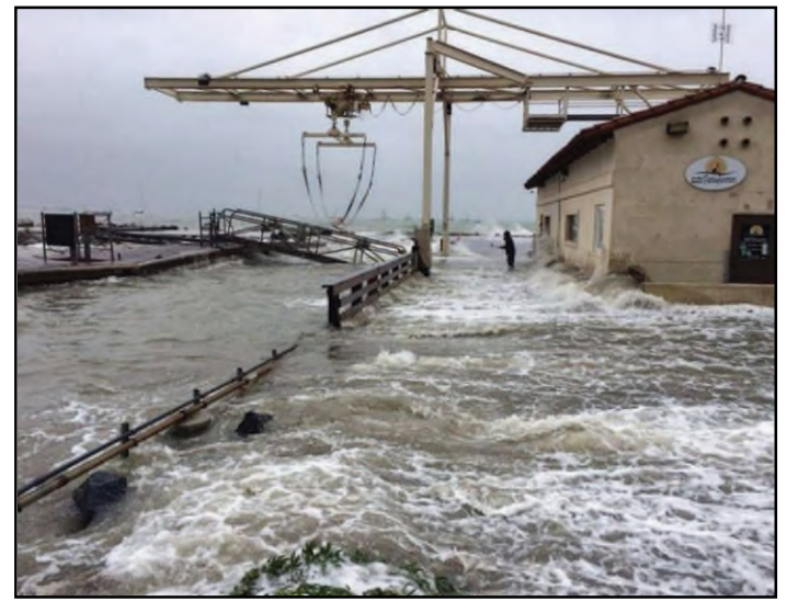
Wave overtopping at the Port San Luis Boat Lift. Photo courtesy of Emily Shay.
