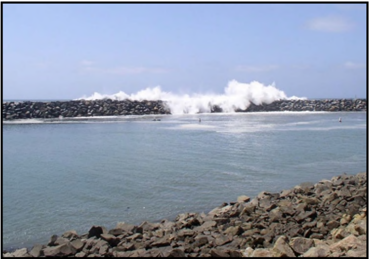
Overtopping of west breakwater (April 2007)
