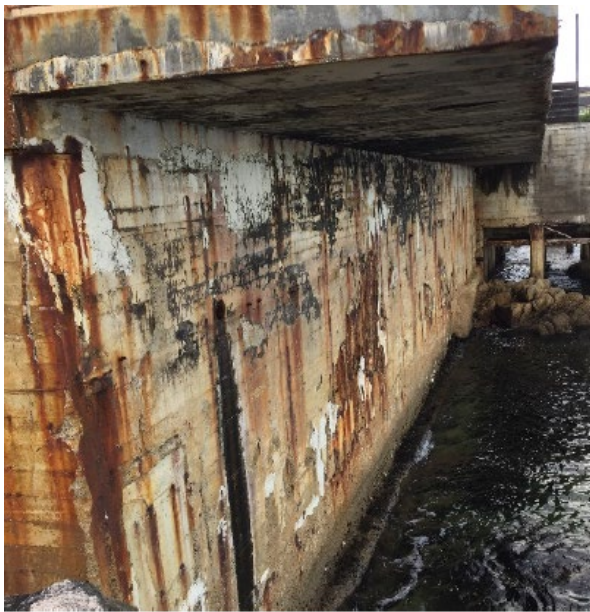
Figure 4: Signs of corrosion and cracking on the Monterey Bay Inn Seawall (City of Monterey)
