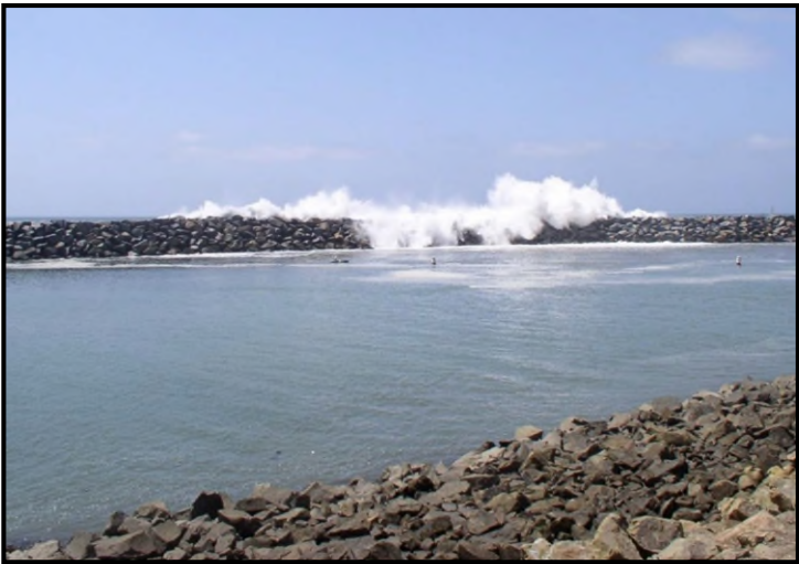
Overtopping of west breakwater (April 2007)
