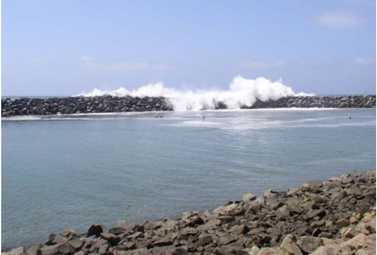
Figure 9: Wave overtopping a breakwater at Dana Point Harbor, April 2007. (Dana Point Harbor)
