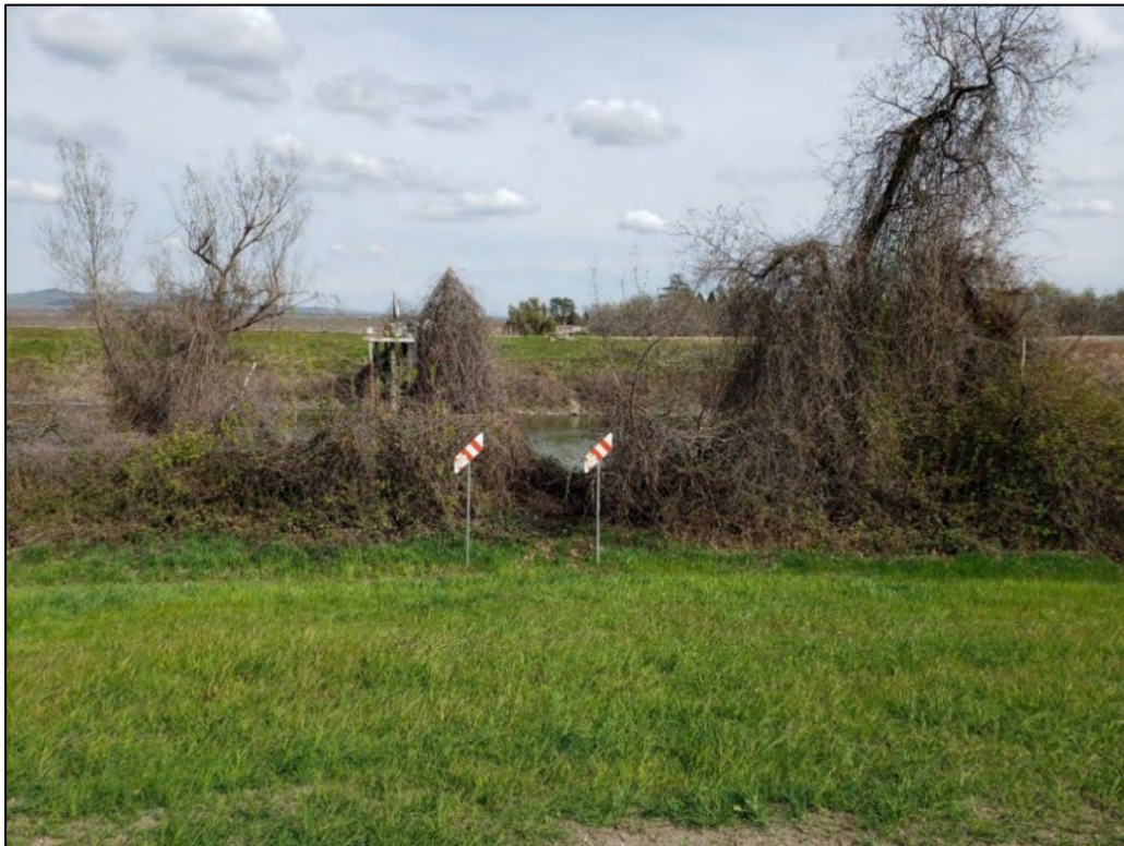
Figure 2-12. Photograph of the Segment 2 Pipeline Alignment on the Waterside Slope of Western Levee
