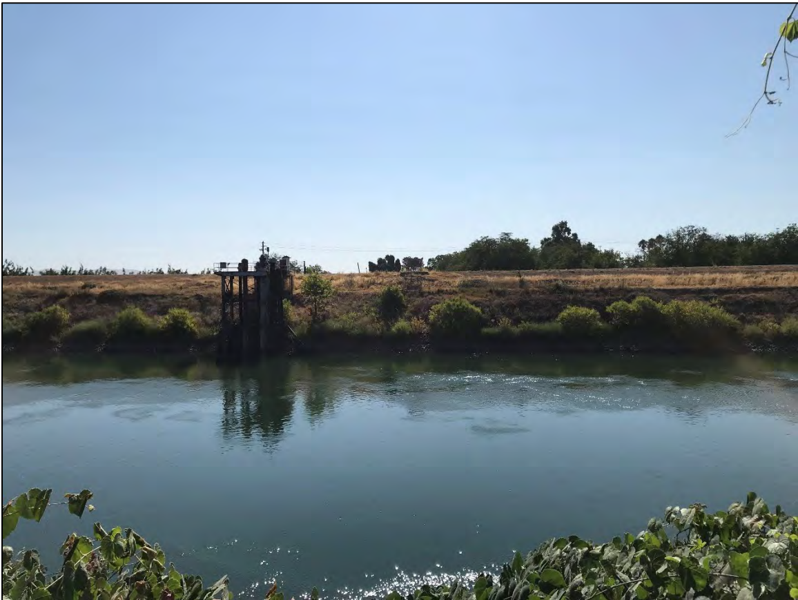
Figure 2-14. Photograph of Segment 4 Pipeline Alignment through East Levee Taken from West Side of Sacramento River
