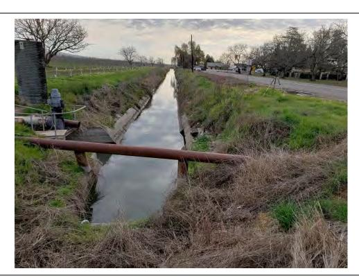
Photograph B. View of marks created by excavation/dredging along the concrete lined agricultural ditch. The flattened pile of dredge spoils can be seen along the top of the bank View southeast (photograph taken 3/17/21).
