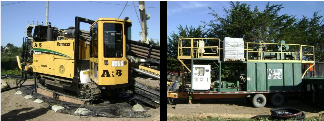
Figure 1. Drill rig placed on timber mats and plastic ground covering with silt fences in the background (left). Separation plant surrounded by straw wattles (right).
