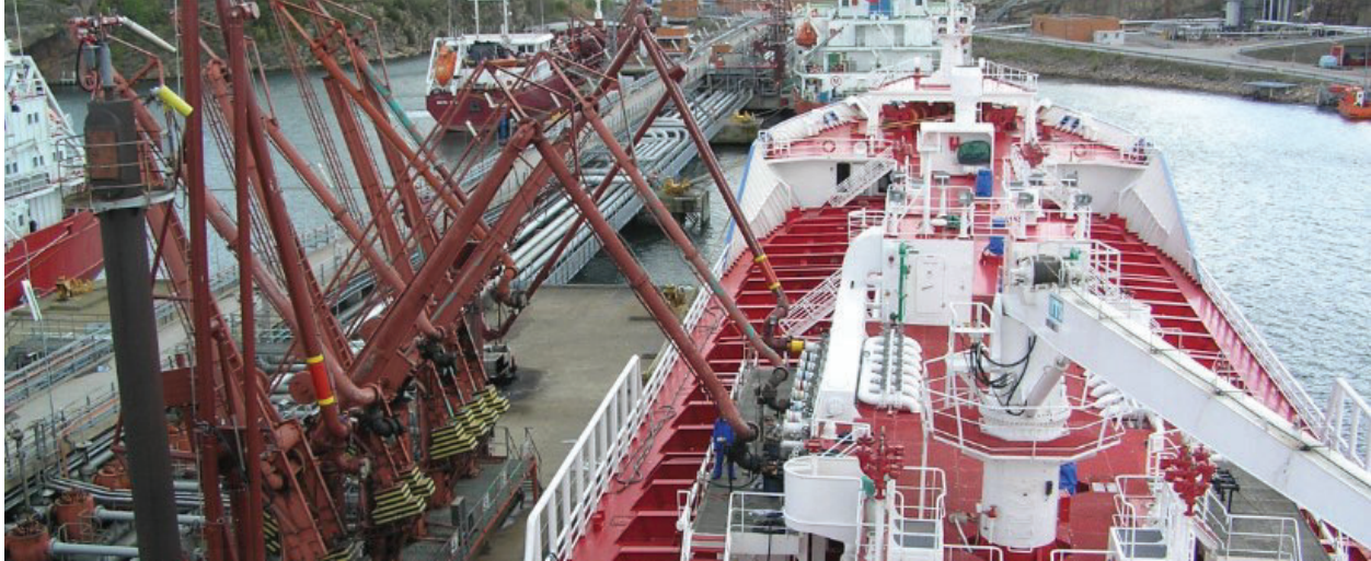
Figure 2 Brofjorden, Sweden marine terminal. Loading arms are similar in size to that needed for SA Recycling’s ballast water handling operations, but smaller than required for Stockton or El Segundo case studies. (source Marcus Bengtsson, wikicommons)
