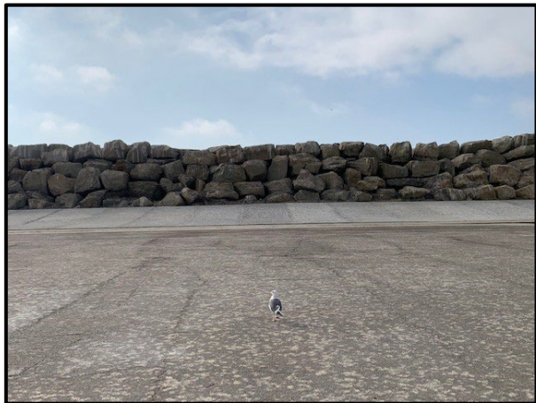
b. Asphalt Leading to Concrete Well Bay Following Completion of Well P&A and Installation of Concrete (Looking South Towards Back of Island Riprap)
