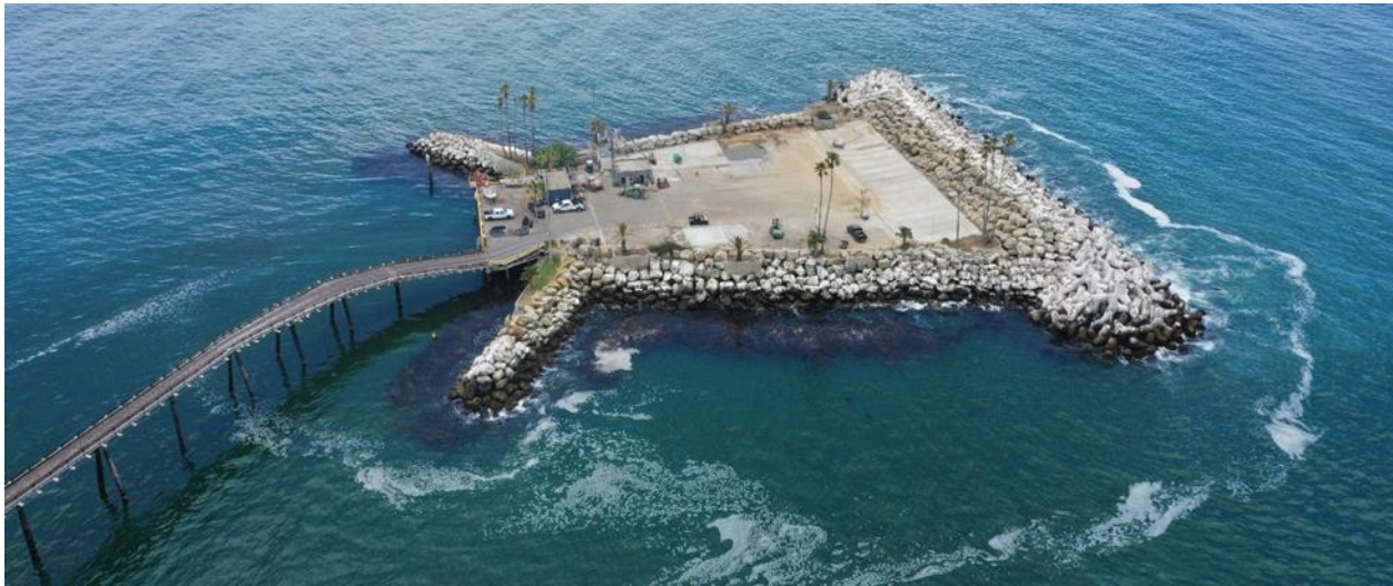
Figure 5 – Aerial Photograph of Rincon Island
