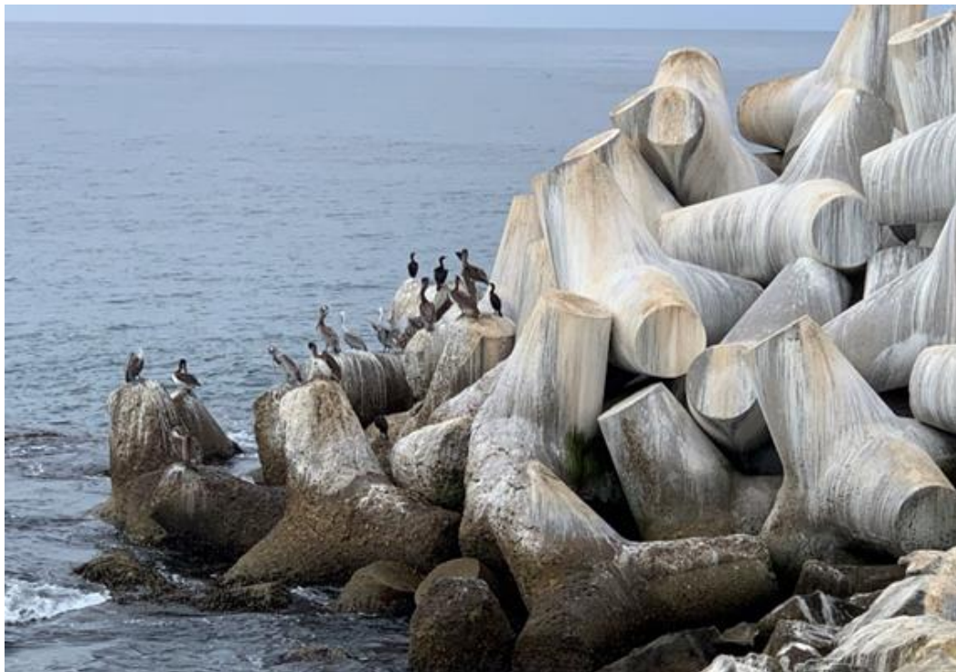
Figure 4 – Concrete Tetrapods
