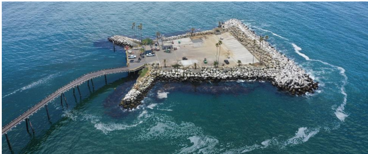
Figure 5 – Aerial Photograph of Rincon Island
