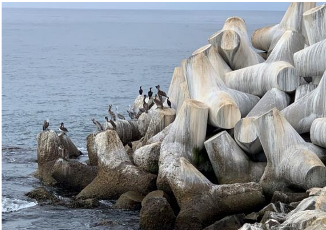
Figure 4 – Concrete Tetrapods
