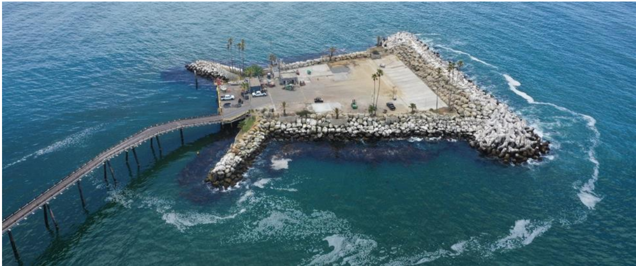
Figure 5 – Aerial Photograph of Rincon Island
