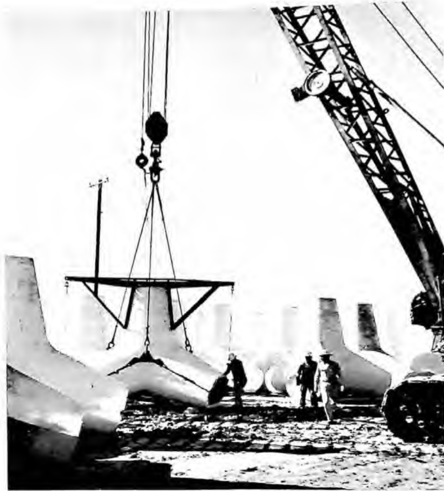
Fig. 14. Handling Tetrapods
