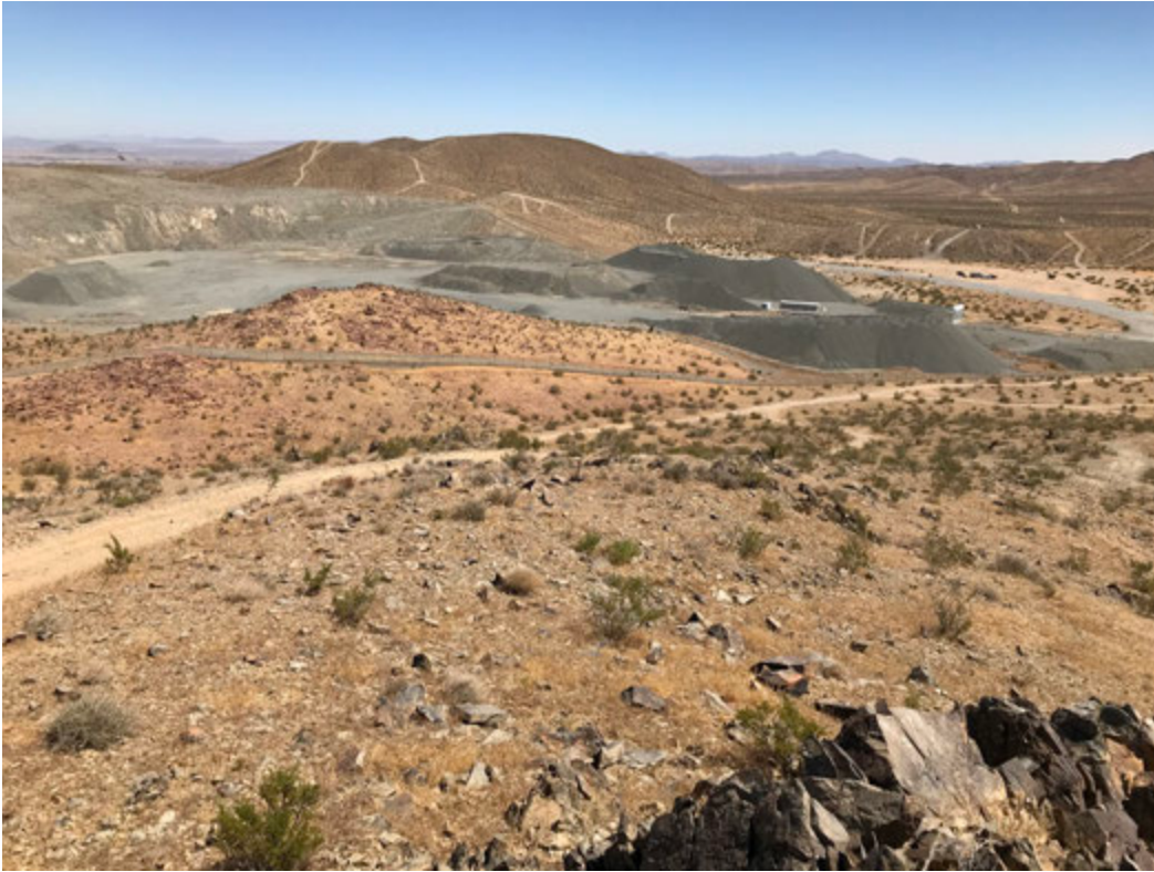
Figure 6: Vulcan Aggregate Quarry and Storage Site.
