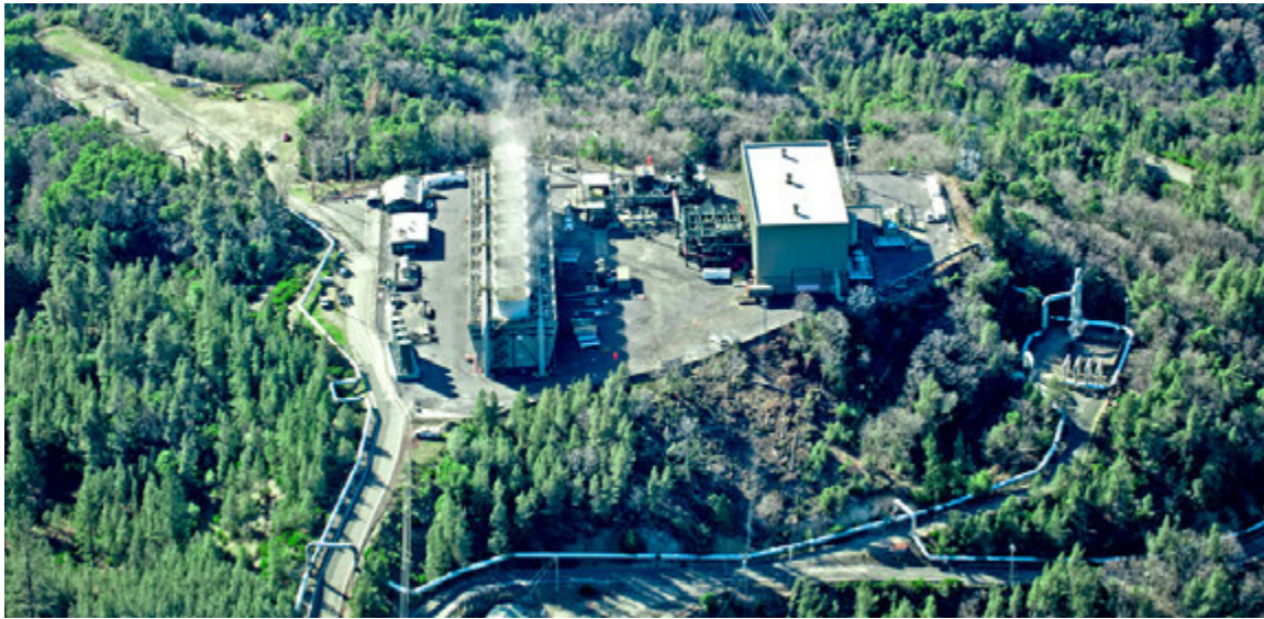
Figure 2: Calpine's Socrates Unit 18 power plant at The Geysers. Photo by John Grice, courtesy of the Calpine Corporation
