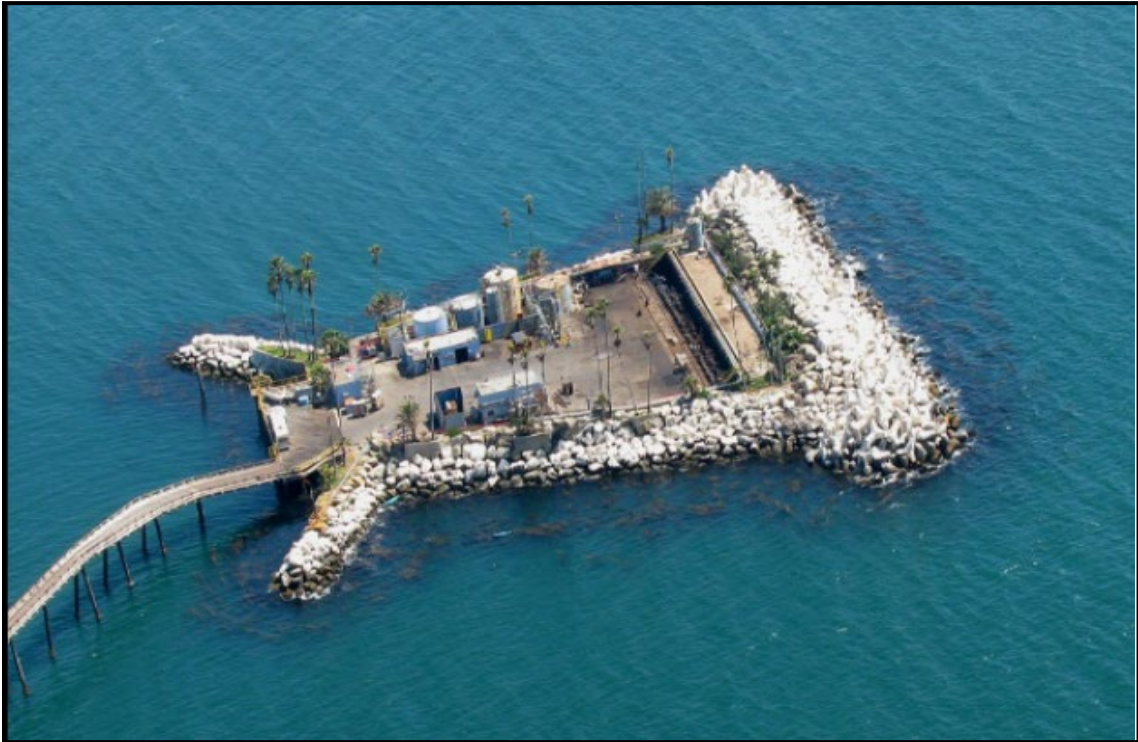
Figure 2. Rincon Island Prior to Phase 1 Decommissioning Activities
