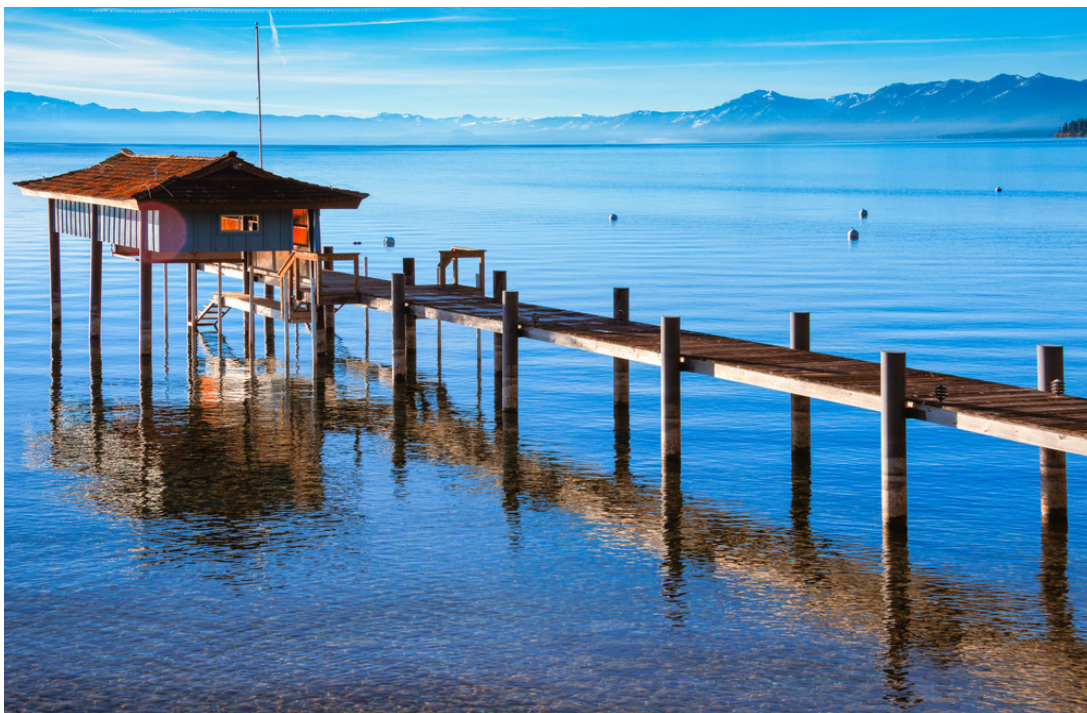
Figure 8: Typical Pier and Boathouse
