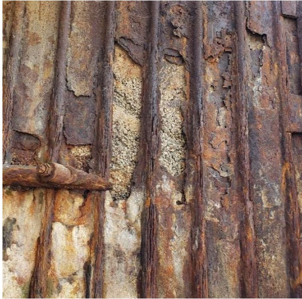
Original Sheet Pile Walls
