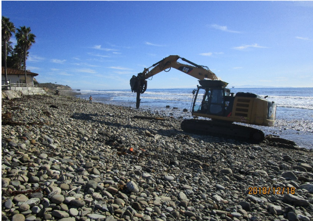
Figure 6. H Beam being extracted near Bacara Resort
