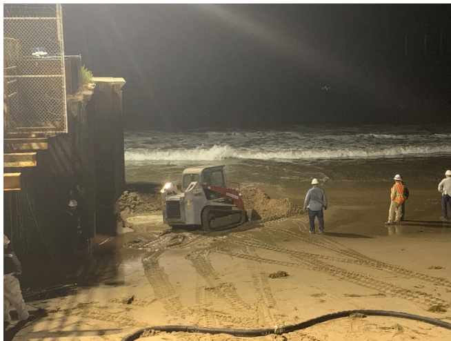
Excavating the Sand Next to the caisson
