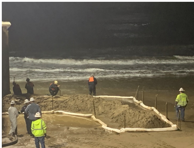
The berm surrounded by oil absorbent boom
