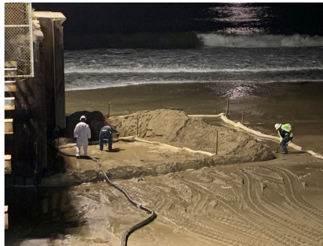
Building the berm around the site of the oil expression on the beach
