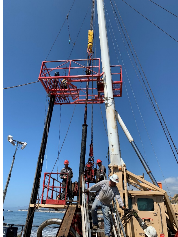
Pulling the Casing
