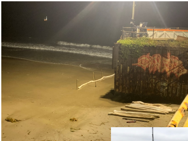
Placement of boom Around caisson
